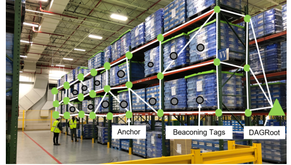
Figure 1: SALT warehouse deployment: shelf anchors form a 6TiSCH mesh, forwarding tag observations to the DAG root.
